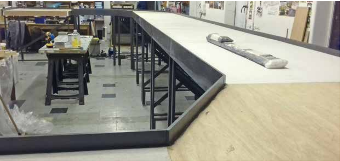
Left The new fiddle yard boards under construction in the Barrowmore MRG clubroom.
